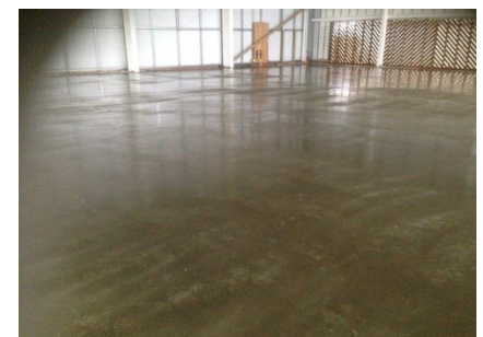
A quality power float finish is easily achieved with the DURUS FLOOR system
