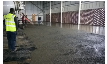
Direct discharge into formwork will reduce construction time
