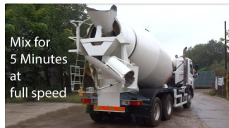
Final 5 minute mix at full speed
