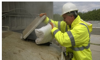
Adding Fibre to the mixer
