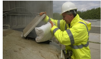
Adding Fibre to the mixer
