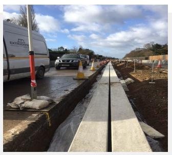
Consistent surface finish is an important factor in this concrete process. The addition of the micro synthetic fibres allows the form to slip more consistently by increasing cohesion and the green tensile strain capacity of the fresh concrete.
