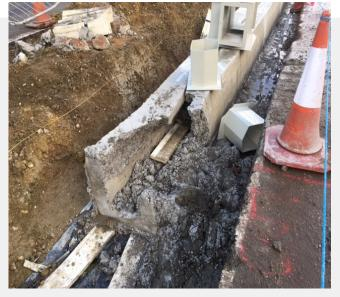
The extruded slot drain can be susceptible to collapse as the profile moves along during installation. The addition of Fibrin XT increases the stability of the fresh concrete, resulting in less defects.
