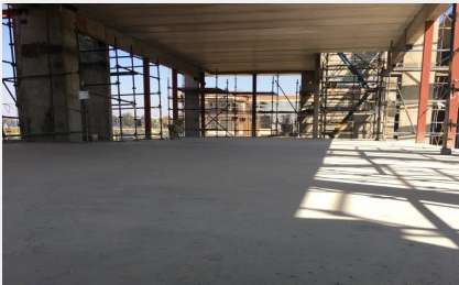
Finished layer of 50mm fibre reinforced screed
