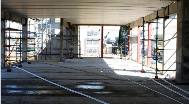
The floor before the Fibre Reinforced Screed was pumped in place
