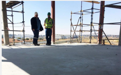
Using monofilament macro fibres allow a nice finish
