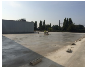
Applying saw cuts within 24 hours
