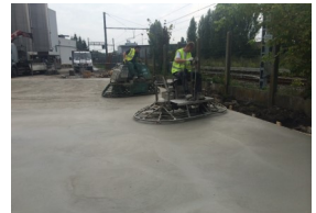
Power floating concrete
