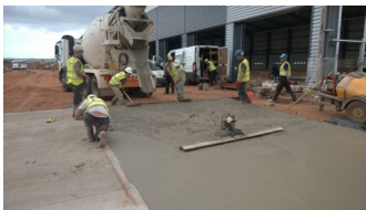
Direct discharge into formwork will reduce construction time
