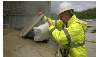
Adding Fibre to the mixer
