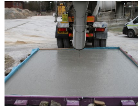
Trail bed being poured
