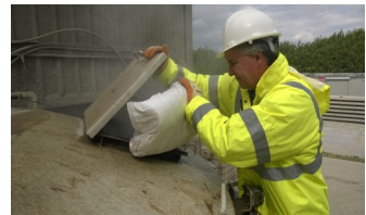
Adding Fibre to the mixer
