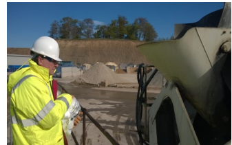
Adding Fibre to the back of the truck
