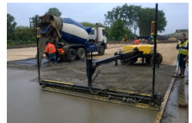
Laser guided screed
