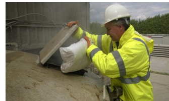
Adding Fibre to the mixer
