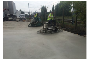
Power floating concrete
