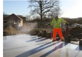
Curing Concrete
