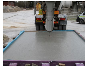
Trail bed being poured
