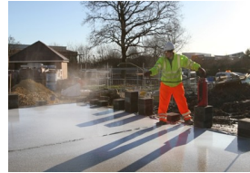
Curing Concrete
