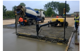
Laser guided screed
