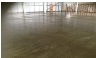
A quality power float finish is easily achieved with the DURUS Floor system
