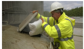
Adding Fibre to the mixer
