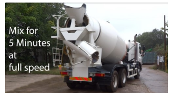
Final 5 minute mix at full speed
