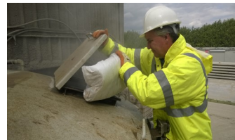
Adding Fibre to the mixer
