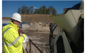
Adding Fibre to the back of the truck
