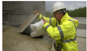
Adding Fibre to the mixer
