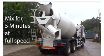
Final 5 minute mix at full speed
