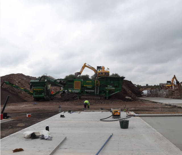
Continuous work during the construction of the slab
