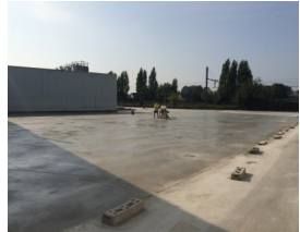
Applying saw cuts within 24 hours
