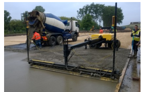
Laser guided screed
