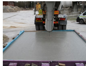
Trail bed being poured
