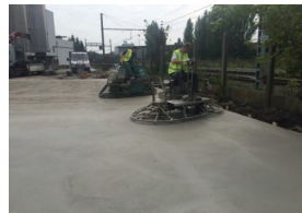
Power floating concrete
