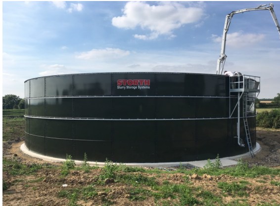
StorTh Slurry Tank Base
