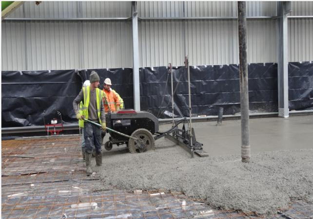
A laser screed could be used continuously without the need for breaks in installation to fix a top layer of conventional steel mesh reinforcement.
