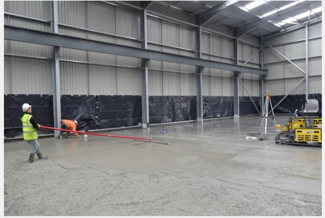
Large areas of pavement could be poured and power floated. Saw cut contraction joints were then made the following day.
