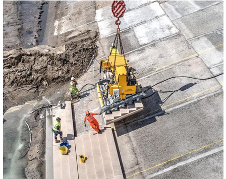
Sea Defence Installation
