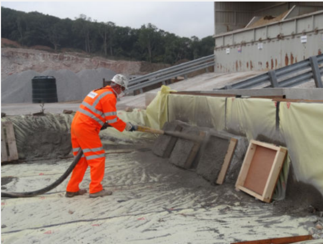
Preparing shotcrete panels for EFNARC Tests
