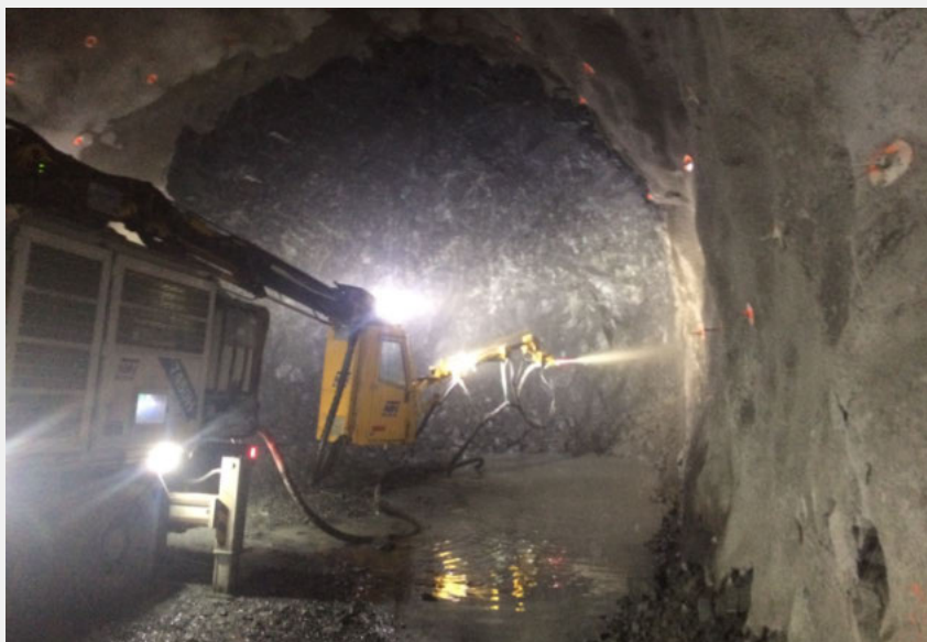
Shotcreting walls after drill and blast
